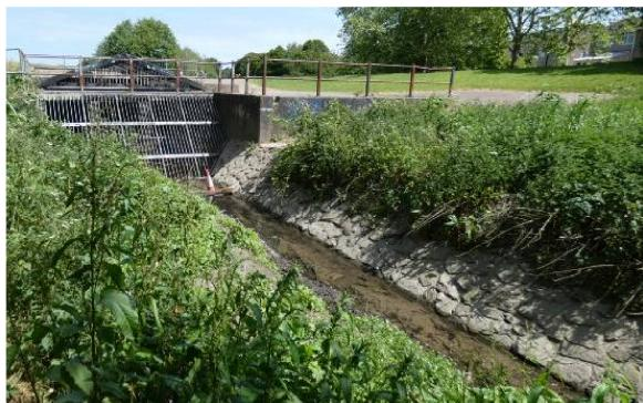
Following a devastating flood in 1968, it was decided to take the Malago's water away from the stream and carry it down a huge culvert to join the New Cut in Southville. The water was intercepted at the large structure we see today. This culverting means that there is no true Malago water in the Malago as it passes through Bedminster and joins the New Cut at Cumberland Basin.
