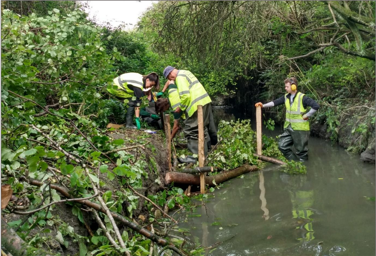
Figure 2. A woody debris berm (type of complex woody debris feature) being created by BART and volunteers in the Stoke Brook.
